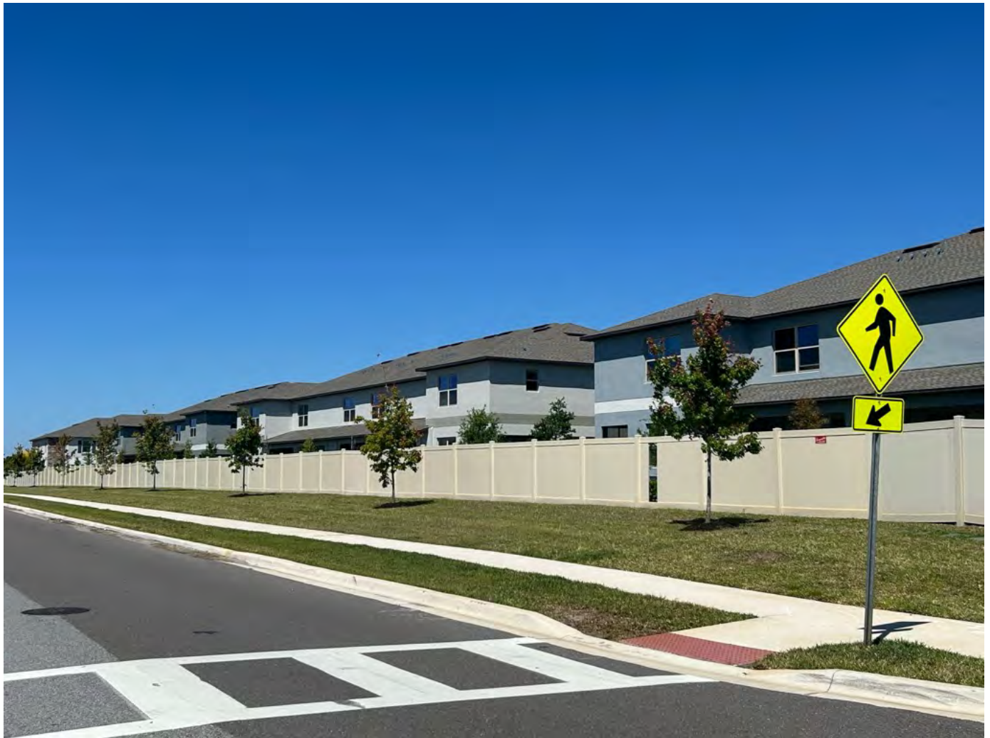
West Common Area- Mowed And Line Trimmed
